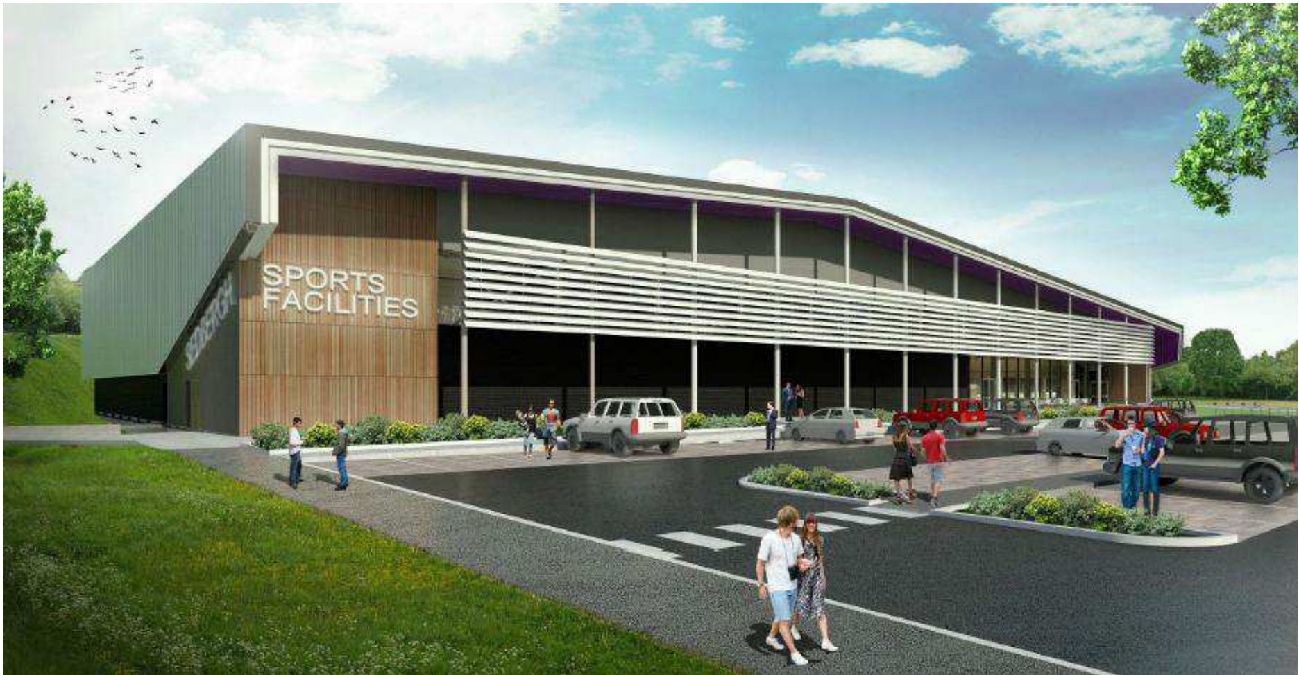
View from South East Corner of car park
